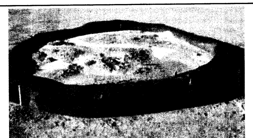
FIGURE 3.18 Typical Compost Sock Washout Installation
